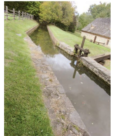
Water traveled from the millpond in the millrace to the distillery and gristmill at Mount Vernon Estate.
